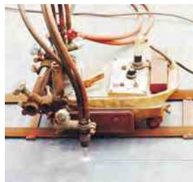
Gas Cutting 气割
